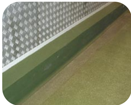
Rendered Concrete Kerb
